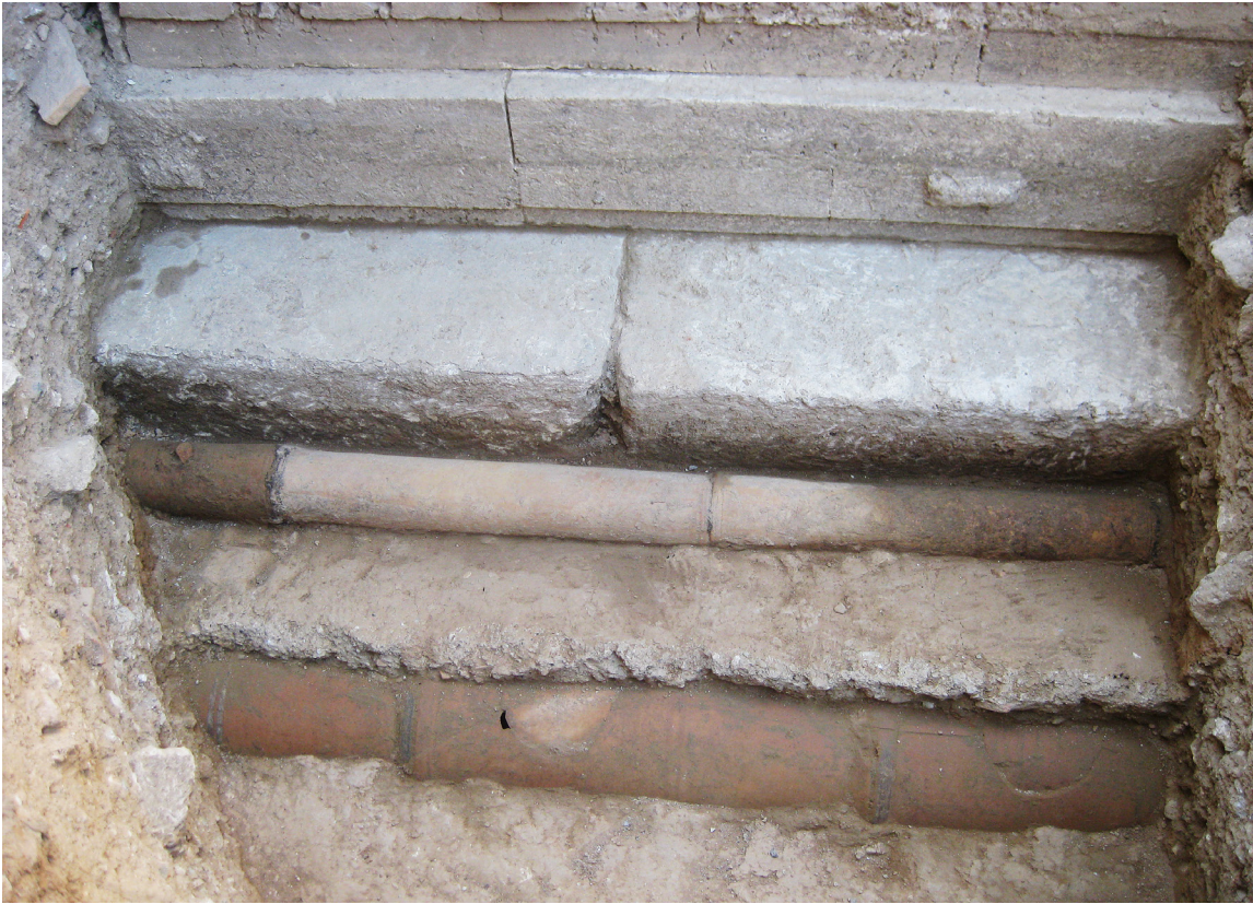
Fig 11 The two terracotta pipelines discovered behind the back wall of the Painted Stoa.
