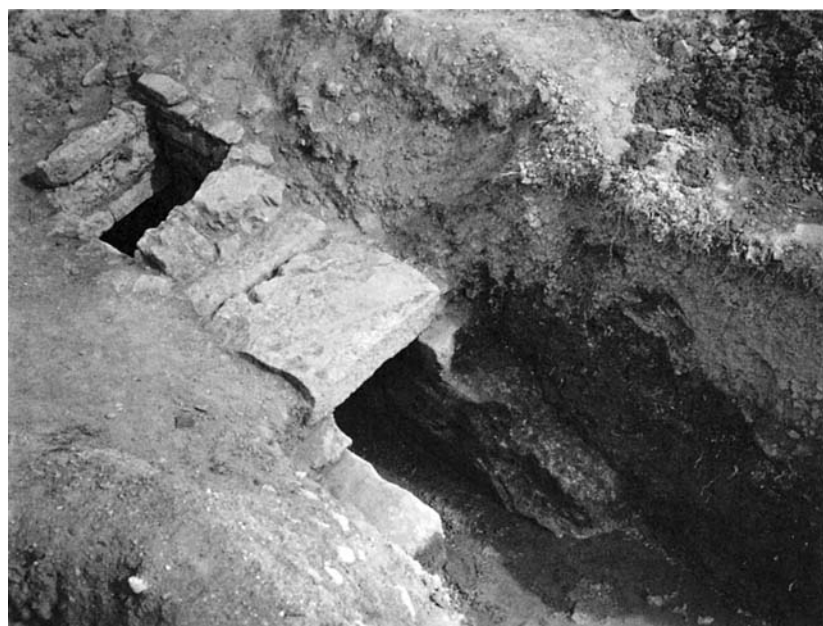
37. Great Drain, East Branch with Manhole.
