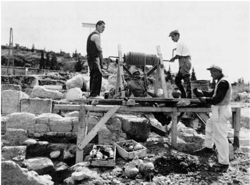
7. Excavating a Well.
