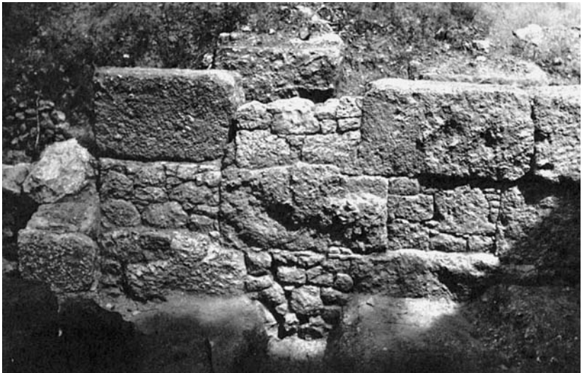
34. Wall of the Great Drain, West Branch.
