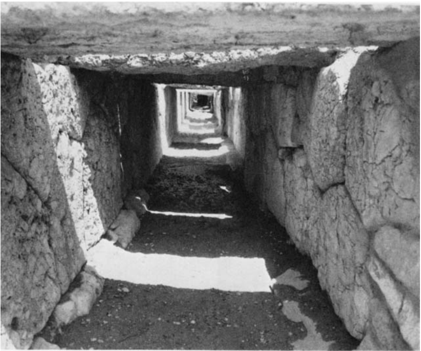
33. The Great Drain of the Agora. Width of Channel one meter.
