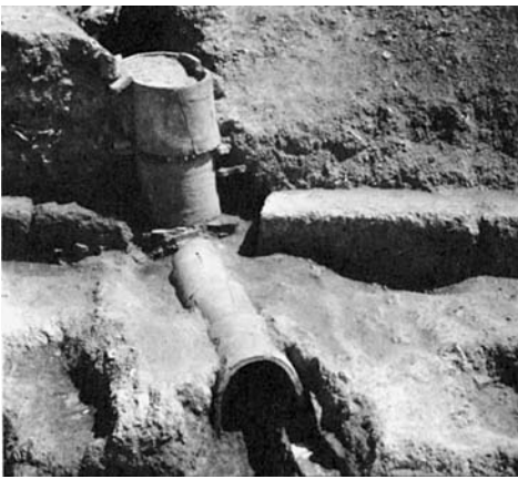
39. Built Drain of Late Roman Period with Manhole.
