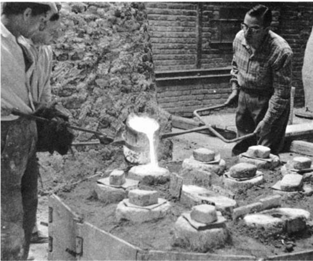
32-34. Lost-wax casting, although now refined in the details, is a process which has not changed significantly since antiquity. These views of a present-day foundry show the building up of a clay mold, a brick furnace much like an ancient one, and the pouring of bronze into funnels leading to molds packed in a makeshift casting pit. 1957.
