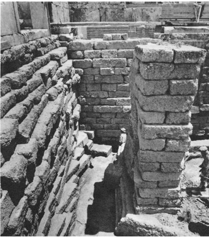
16. Conglomerate foundations of the Stoa of Attalos, ca. 150 B.C. The pier at the right, 17 courses deep, supported one of the columns of the interior colonnade.
