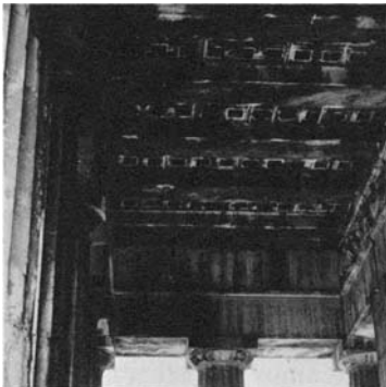
36. Coffered ceiling, east porch of the Hephaisteion.
