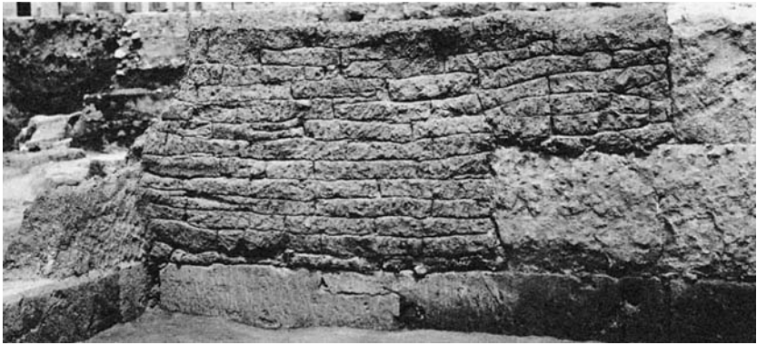
10. Mud-brick walls resting on stone orthostates, with a floor of packed clay. South Stoa I, 430–420 B.C.
