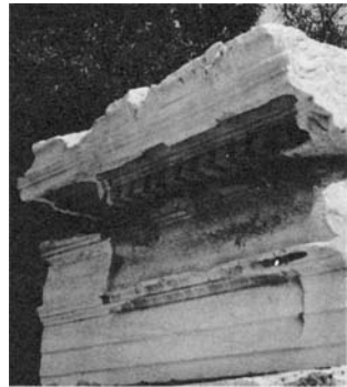
34. Ionic entablature of the Southeast Stoa, Roman period, showing the use of dentils. Note also that frieze and architrave are carved from a single block.
