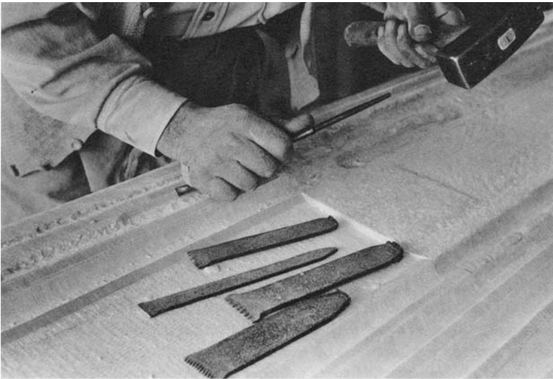
15. A selection of chisels used in the reconstruction of the Stoa of Attalos.
