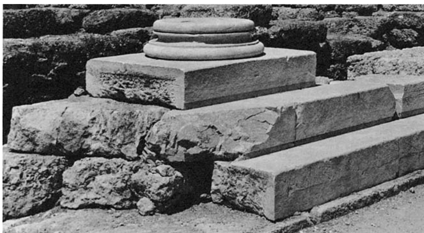
8. Steps of the Metroon, 2nd century B.C. The Ionic column base is of white Pentelic marble, the steps of blue Hymettian marble, and the foundations of hard, gray limestone. The step block below the column base displays the usual treatment of a joint surface ( anathyrosis ).
