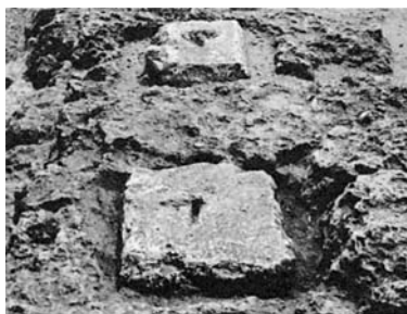
8. Steps of the Metroon, 2nd century B.C. The Ionic column base is of white Pentelic marble, the steps of blue Hymettian marble, and the foundations of hard, gray limestone. The step block below the column base displays the usual treatment of a joint surface ( anathyrosis ).
